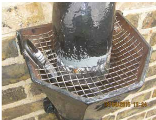
Rainwater downpipe overflow/blockage sensor.
