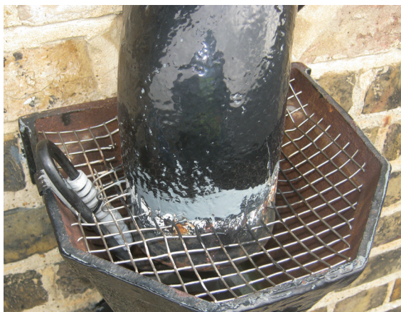
Rainwater downpipe overflow/blockage sensor.
